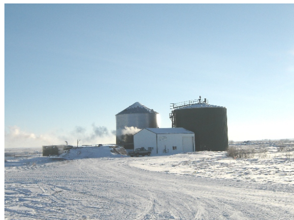
AD system operates efficiently through the winter months on a 1200-sow farrow-to-finish operation near Saskatoon, SK
