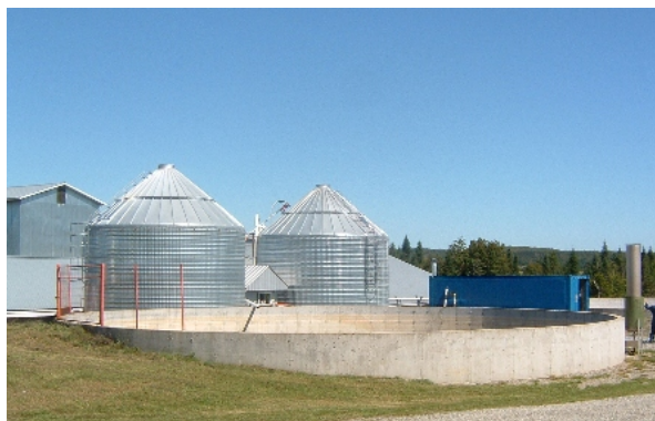
Anaerobic digestion system on 170 sow farrow-to-finish operation in Sherbrooke, QC
