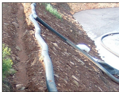
Figure 2. Plastic perforated tile and burial trench.
