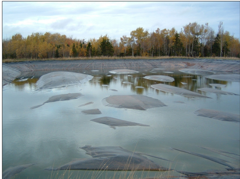
Figure 1. Installed NAP cover with precipitation water on surface.
