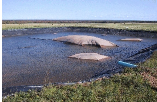
Negative air pressure cover for earthen manure storage.
